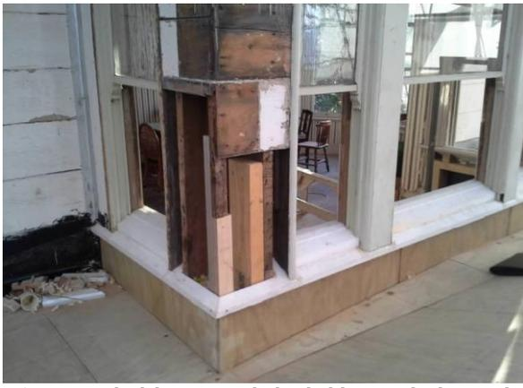
1. Removal of the external ply cladding to the bay and surrounding elevation has revealed the old weatherboards and timber quoins
