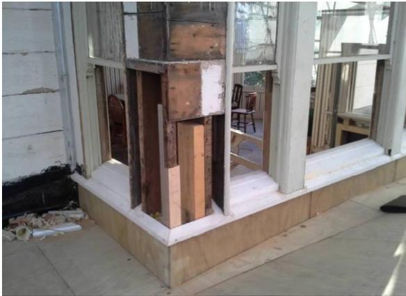
2. The lower sashes to the bay have been sent away for re-sizing and new sills to the bay have been installed.
