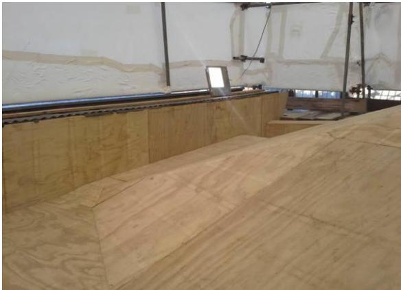
3. The ply diaphragm has been extended across the whole of the 1960s octagonal roof and the surrounding flat roofs and new internal gutters have been formed.
