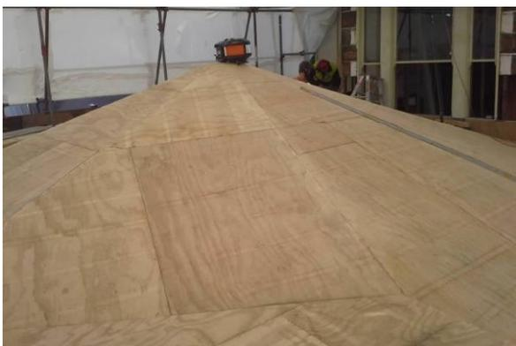
4. The ply upstand to the 1964 roof has been constructed and the inside face/top of the block parapet wall has been clad.
