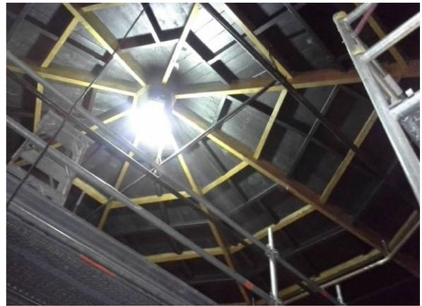
5. The Friends have painted the underside of the roof where visible within the theatre – save for the principal octagon structure, which will remain unpainted (as it was before).
